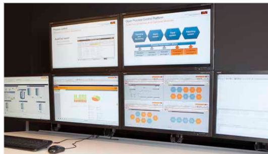
The entire complex in Eggelsberg, with a total of 10,000 data points, is automated by B&R's APROL process control system.
